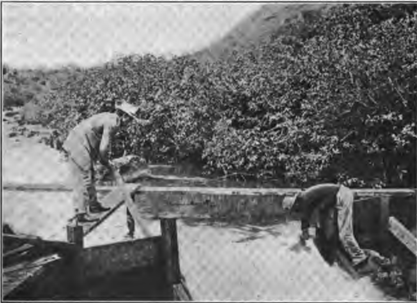
FIG. 20a.—Stream gauging in the Hawaiian Islands.
